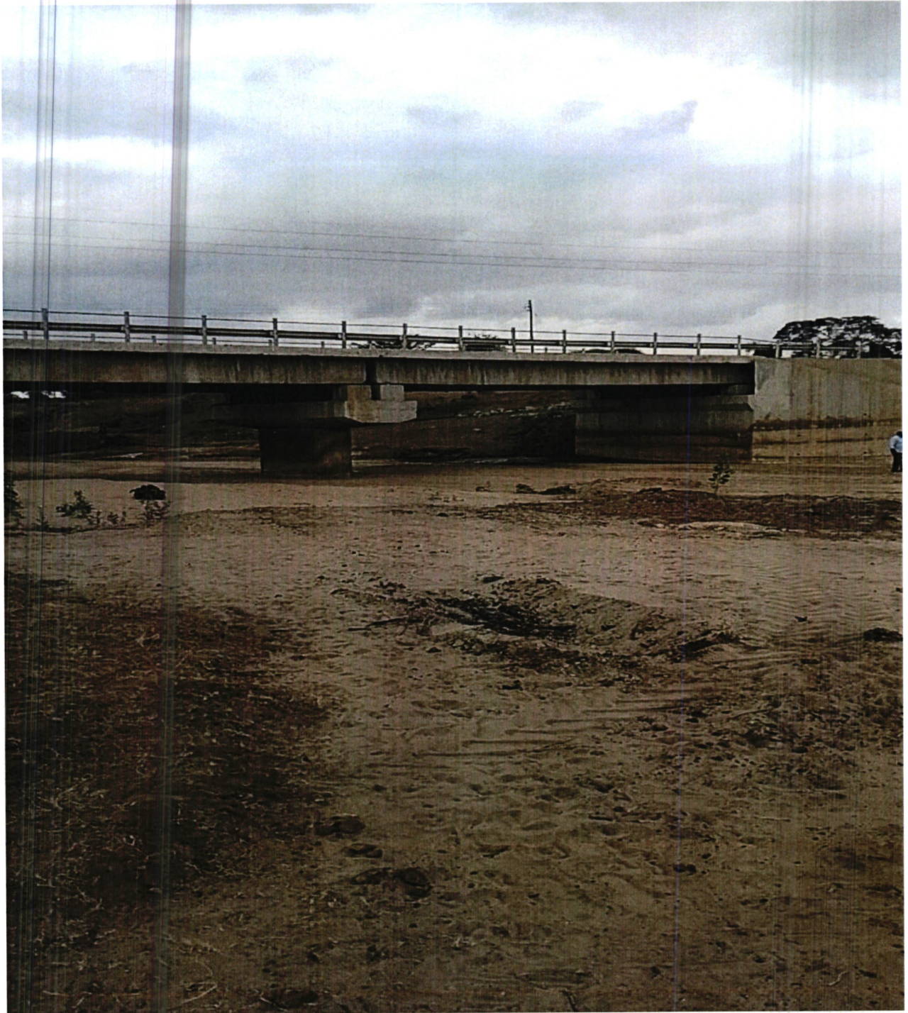
PAII Bridge in Kajiado East connecting Agricultural produce with the Market
