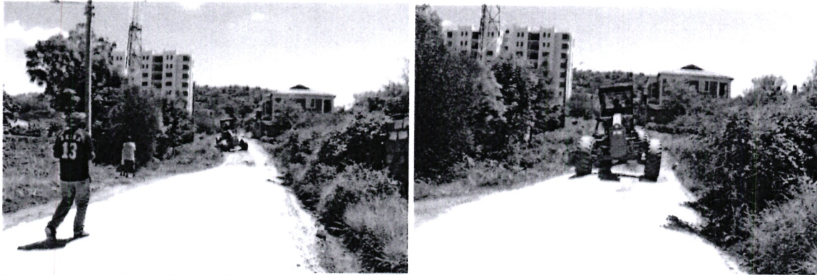
Murraming of Mwakingali roads in Mbololo Ward, Voi sub-county
