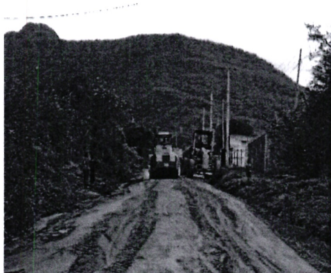
Murraming of Kaloleni feeder roads in Voi.
