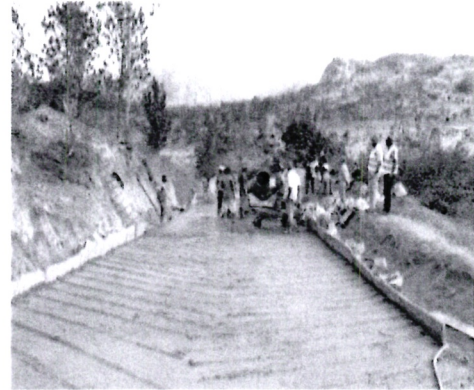
Expansion, grading and slabbing of Kese –Mzazala-Saghasa road in Werugha Ward, Wundanyi sub-county.
