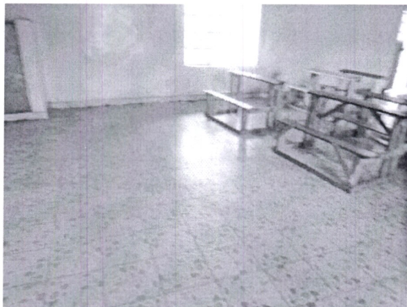
Project name: Kobil primary school Activity: Renovation of 4 classrooms
