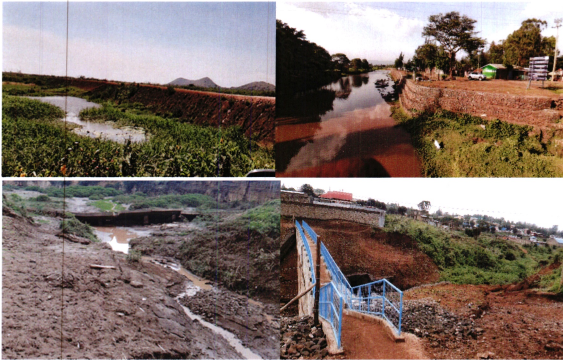
Top left- rehabilitated dyke in Bunyala; top right-gabions along river Nyando banks; bottom left-old Olopito check dam, Narok; bottom right-newly constructed Olopito check dam
