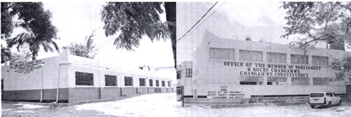
NGCDF Office Block & Gome Primary Laboratories
