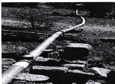
Figure 5: Bulesa to Goda water pipeline extension 3.4 km
