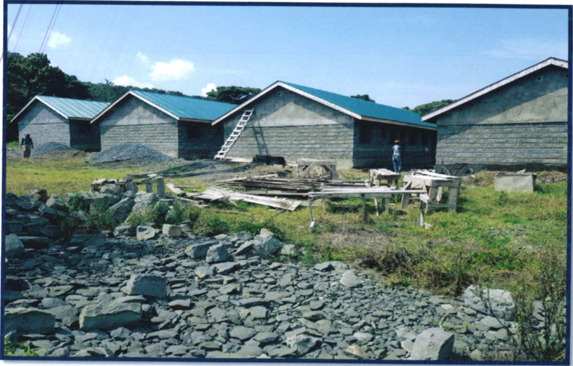
Naivasha Maximum and Women prisons: Completed Staff houses
