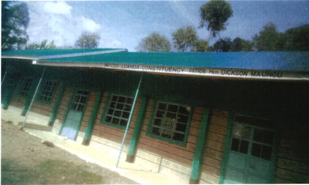
Project 1: Ebbiba Primary school: renovation of 2 No classrooms
