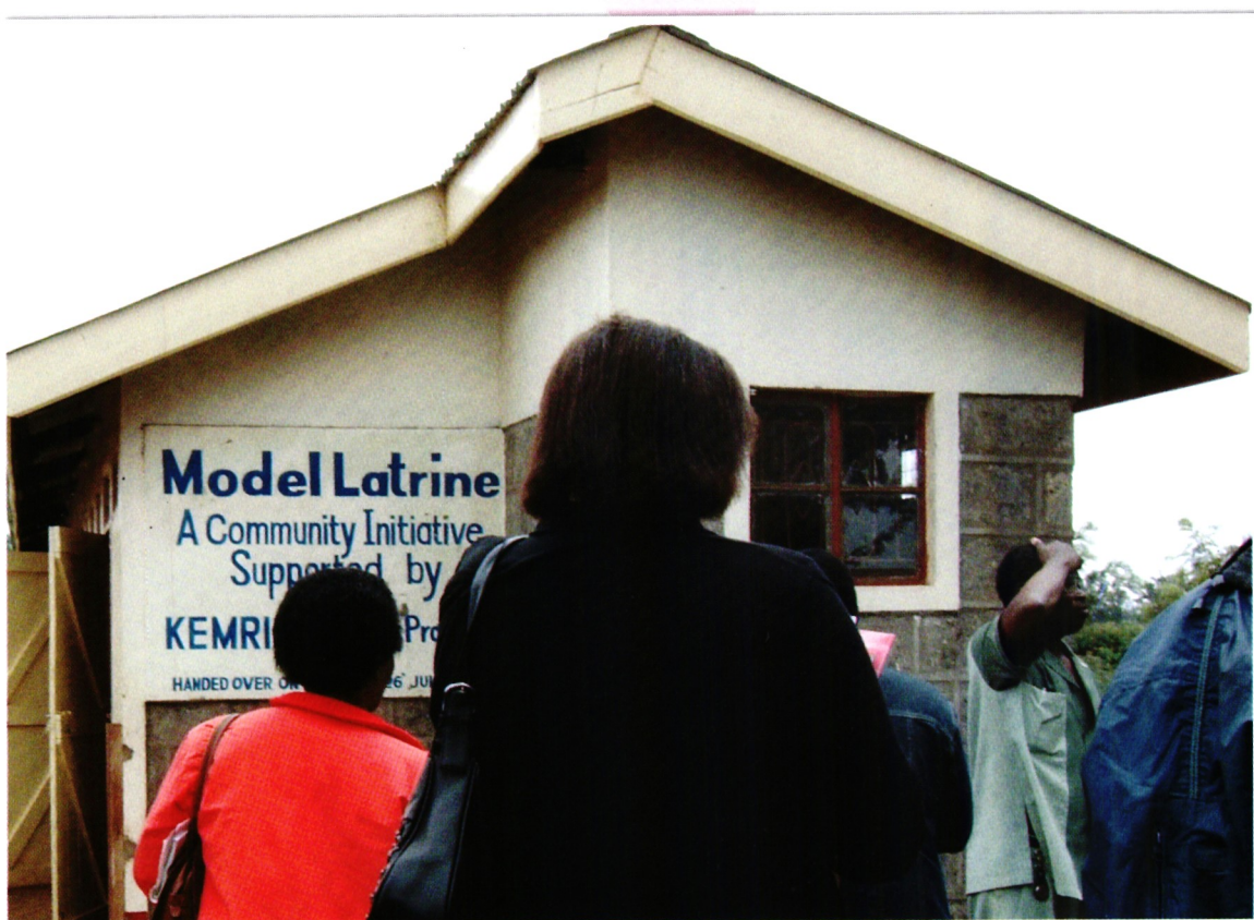
Model latrine constructed through a community initiative with the support of KEMRI/ESACIPAC project under the Mwea School Based Parasite Control Programme
