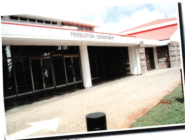
KEMRI Production Facility
