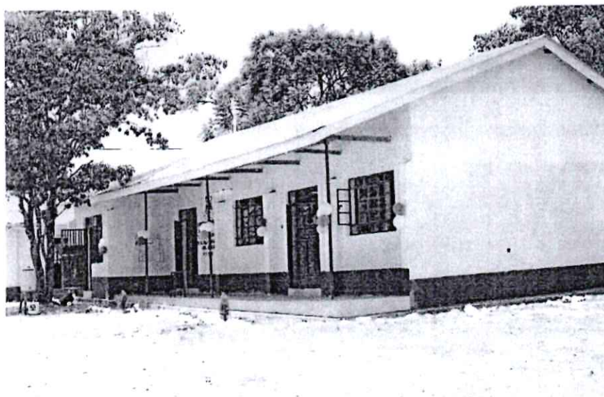
Figure 5: Construction of Science laboratory at St. Sylvesters Girls Secondary School-Madiany
