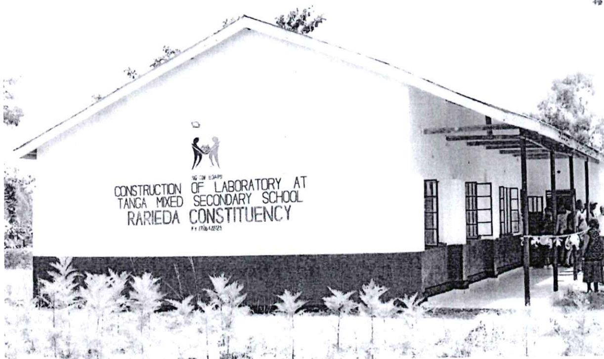
Figure 9: Completion of Construction of laboratory at Tanga Mixed Secondary School
