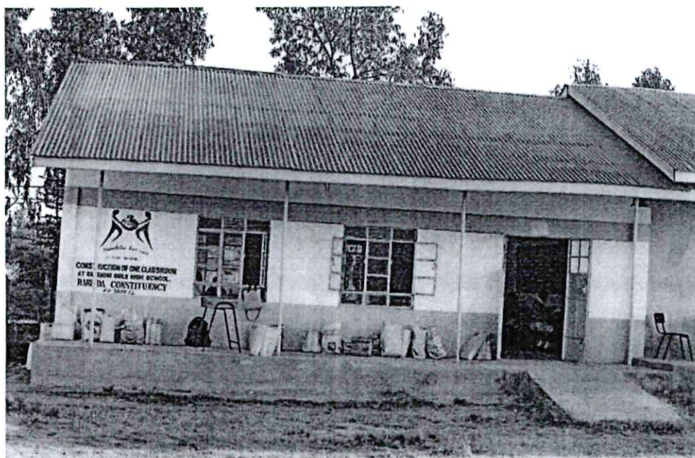
Figure 7: Completion of Construction of one classroom at Rageng'ni Girls High School
