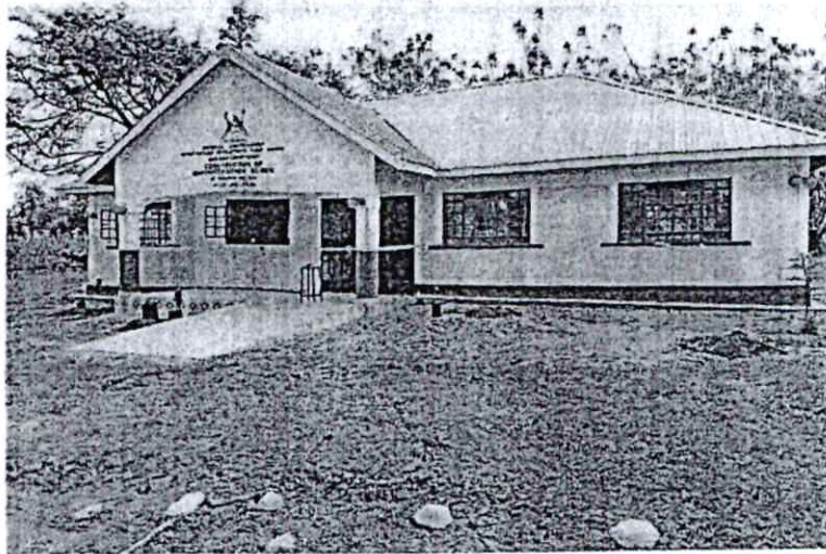
Figure 2 Construction of Administration Block at Mahaya Secondary School
