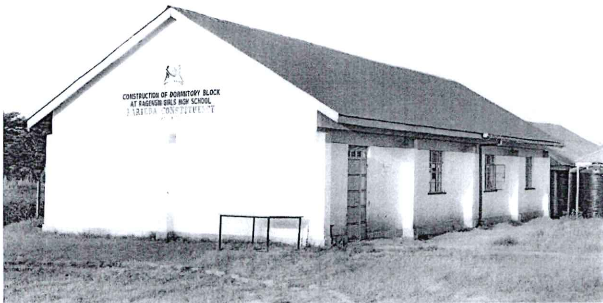
Figure 6: Completion of Construction of Dormitory block at Rageng'ni Girls High School
