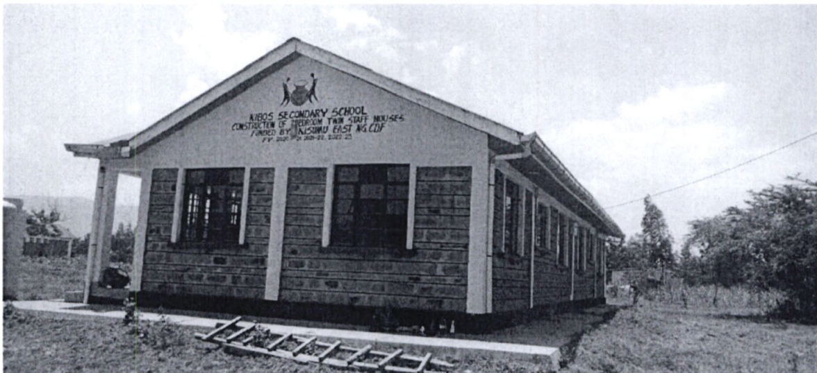
5.construction of two bedroom twin staff houses at Kibos secondary school
