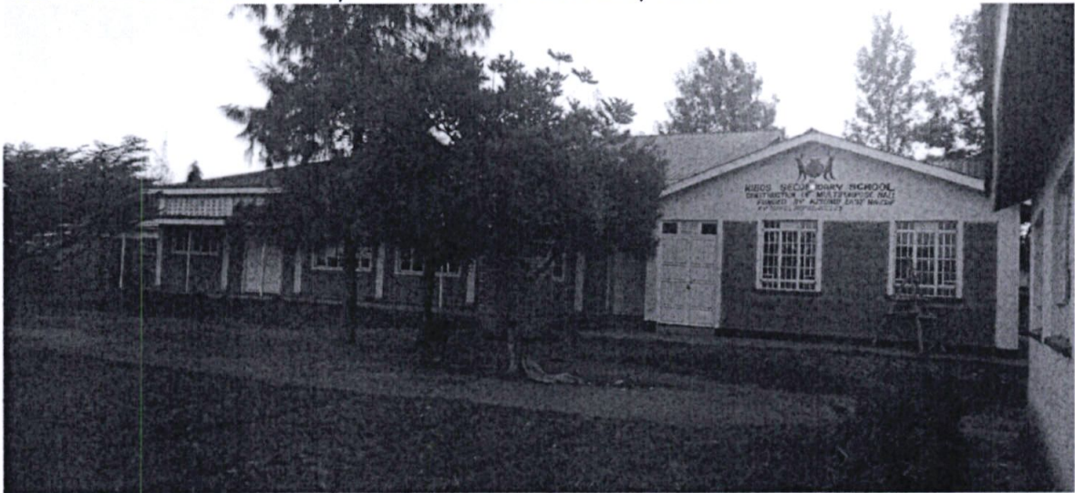
3.construction of a multipurpose hall at kibos secondary school
