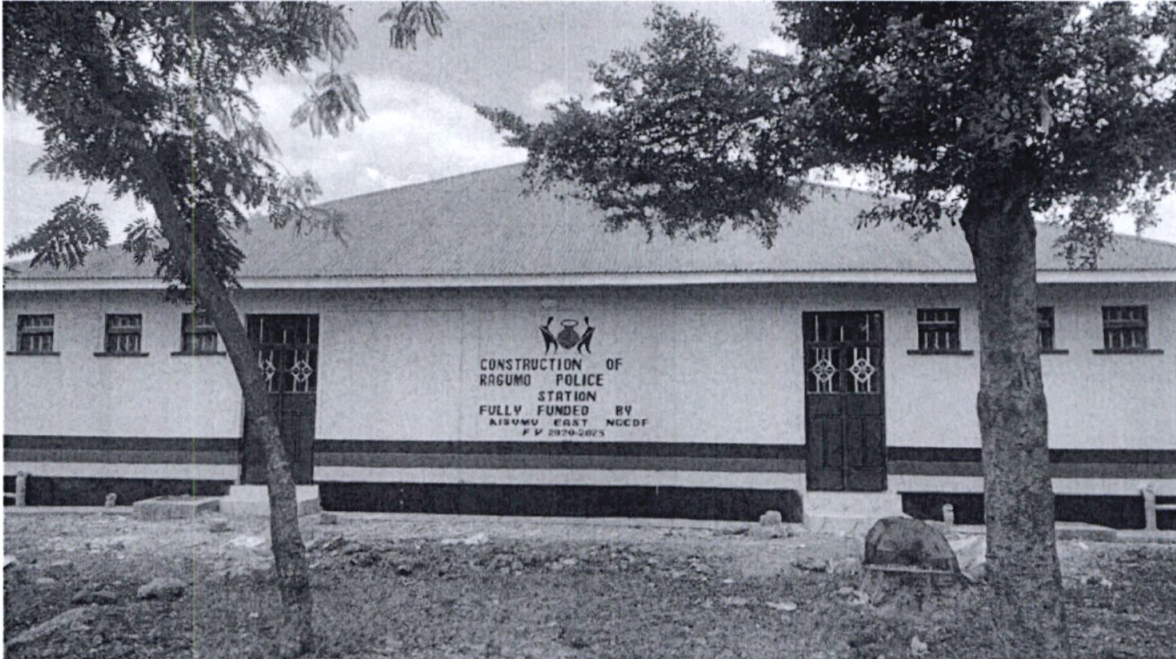
4.construction of ragumo police station
