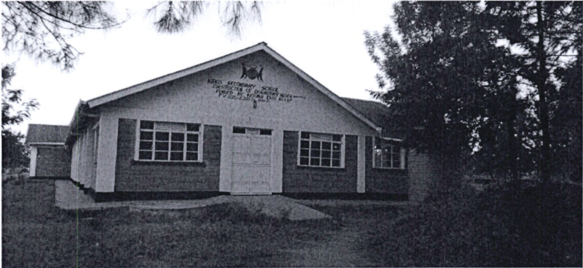
2.consruction of a dormitory block at kibos secondary school
