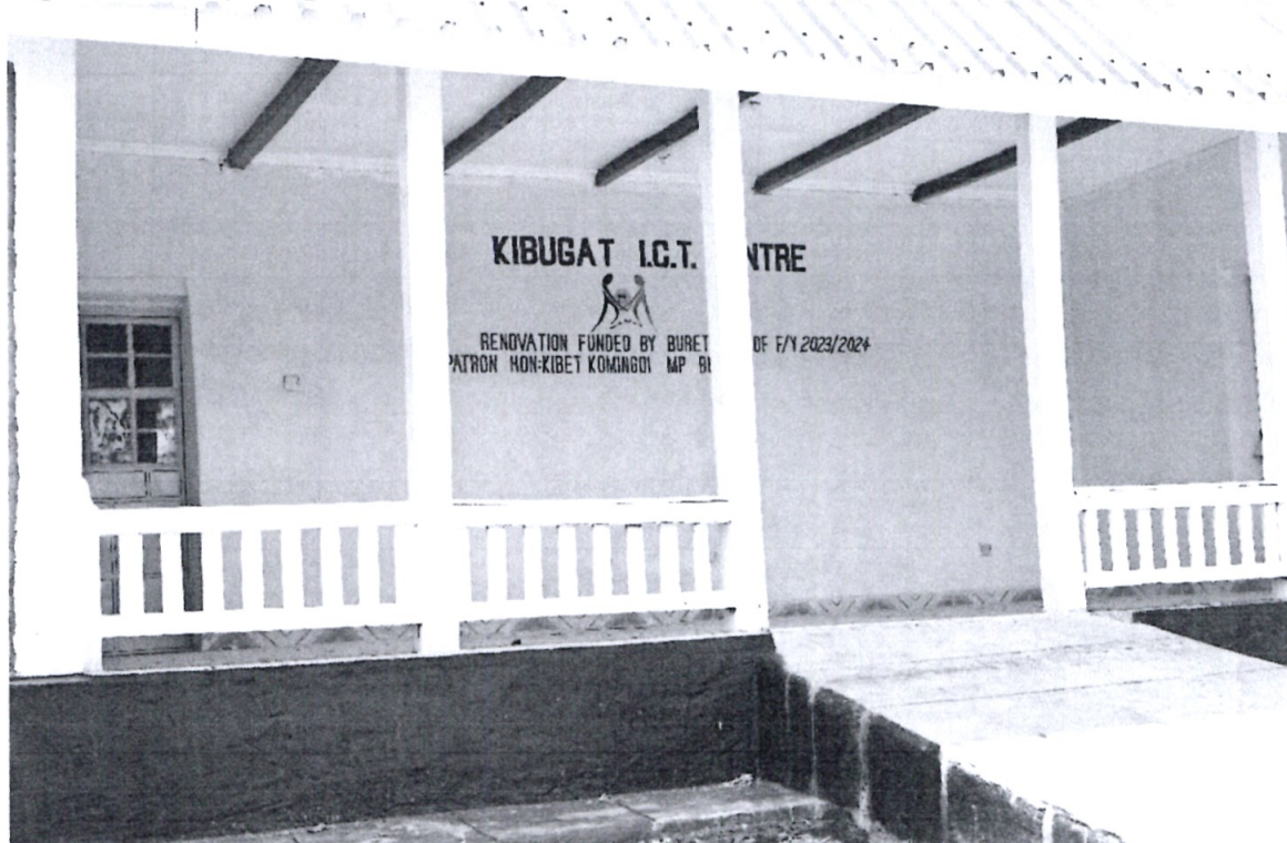
Fig 1.6: Photo of completed renovated ICT Center at Kibugat
