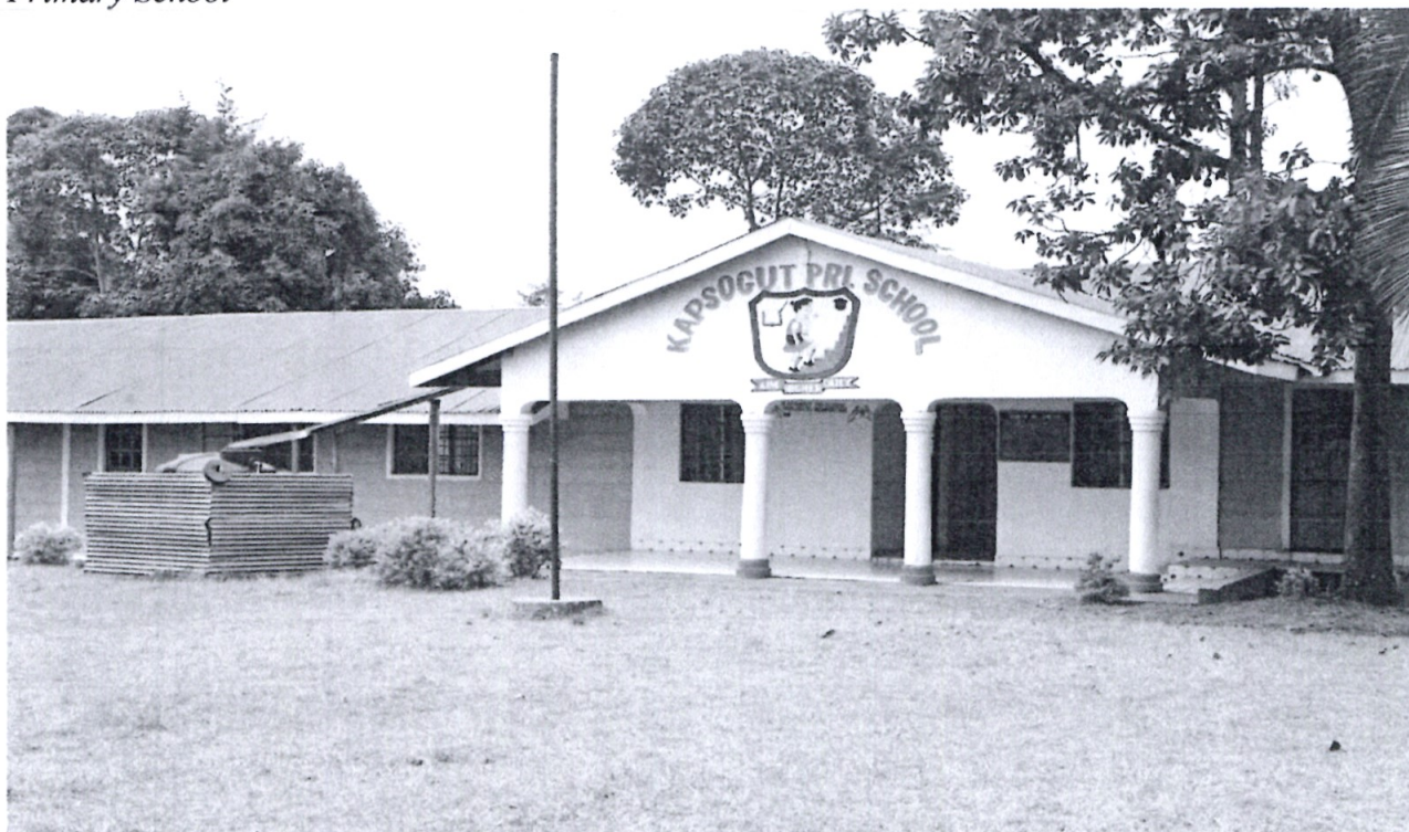
Fig 1.5 Photo of completed 13 renovated classrooms at Kapsogut Primary School
