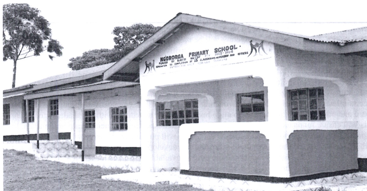
Fig 1.7: Photo Of Completed 15 Renovated Classrooms, Workshop And Offices At Ngororga Primary School
