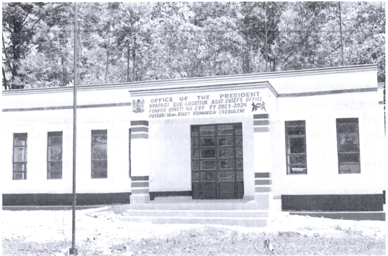
Fig 2; Photo Of Completed Chief's Office At Mabasi location.
