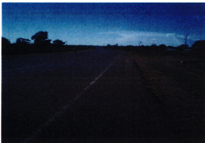
Picture 4: Completed road- Bondo-Misori road (August 2014)
