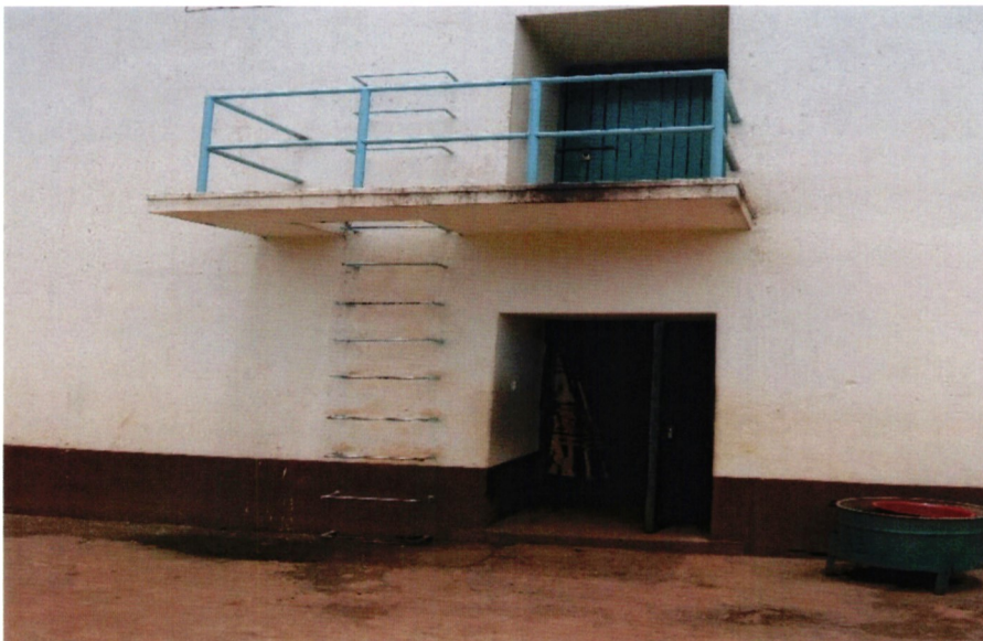
Source: Physical verification of firefighting equipment by OAG Staff
