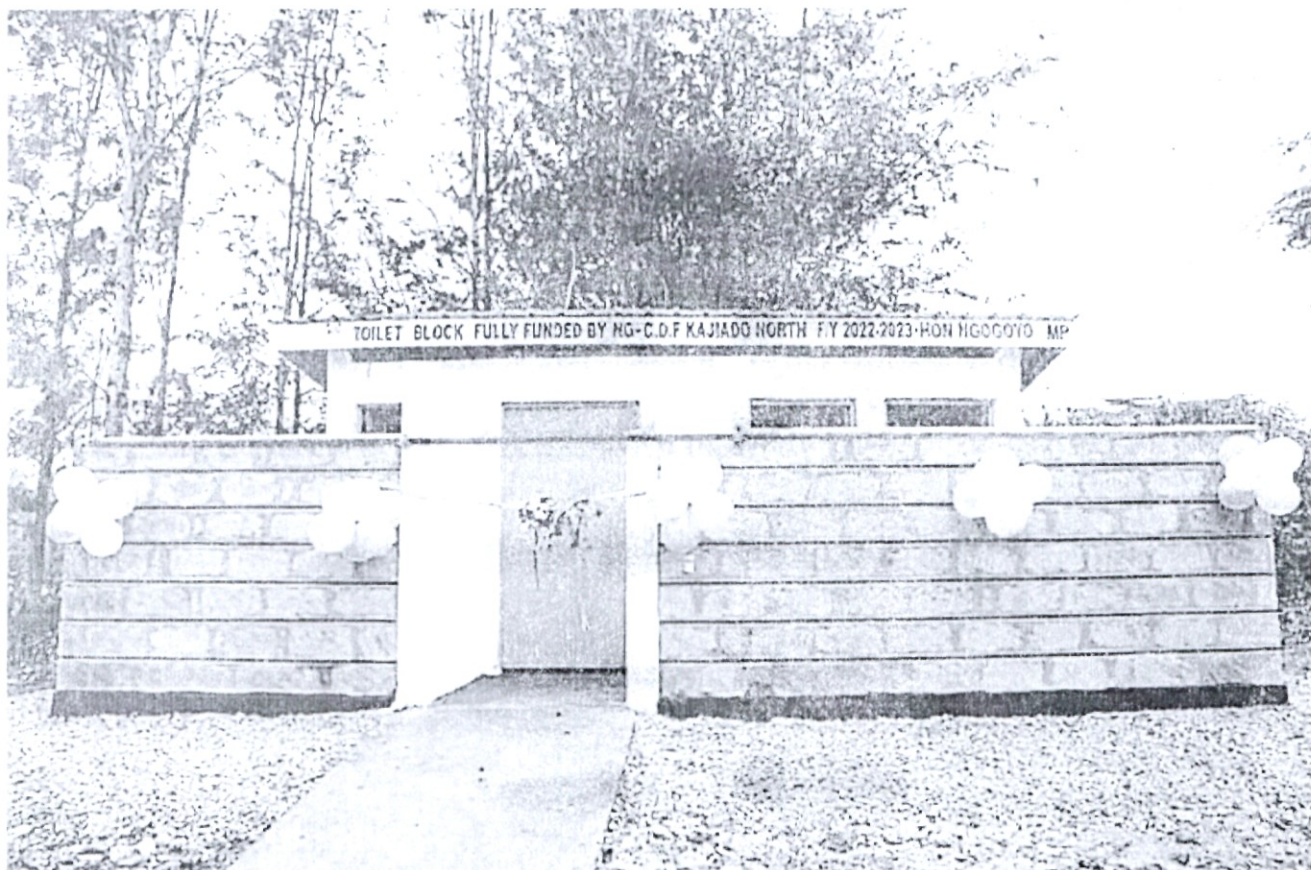
Staff Toilet at Enoomasiani Mixed Day Secondary School. Impact: Facility useful to the 33 staff members of the school with the principal who is PLWD thereby translating to impact on the approximately 1300 students enrolled in the school.
