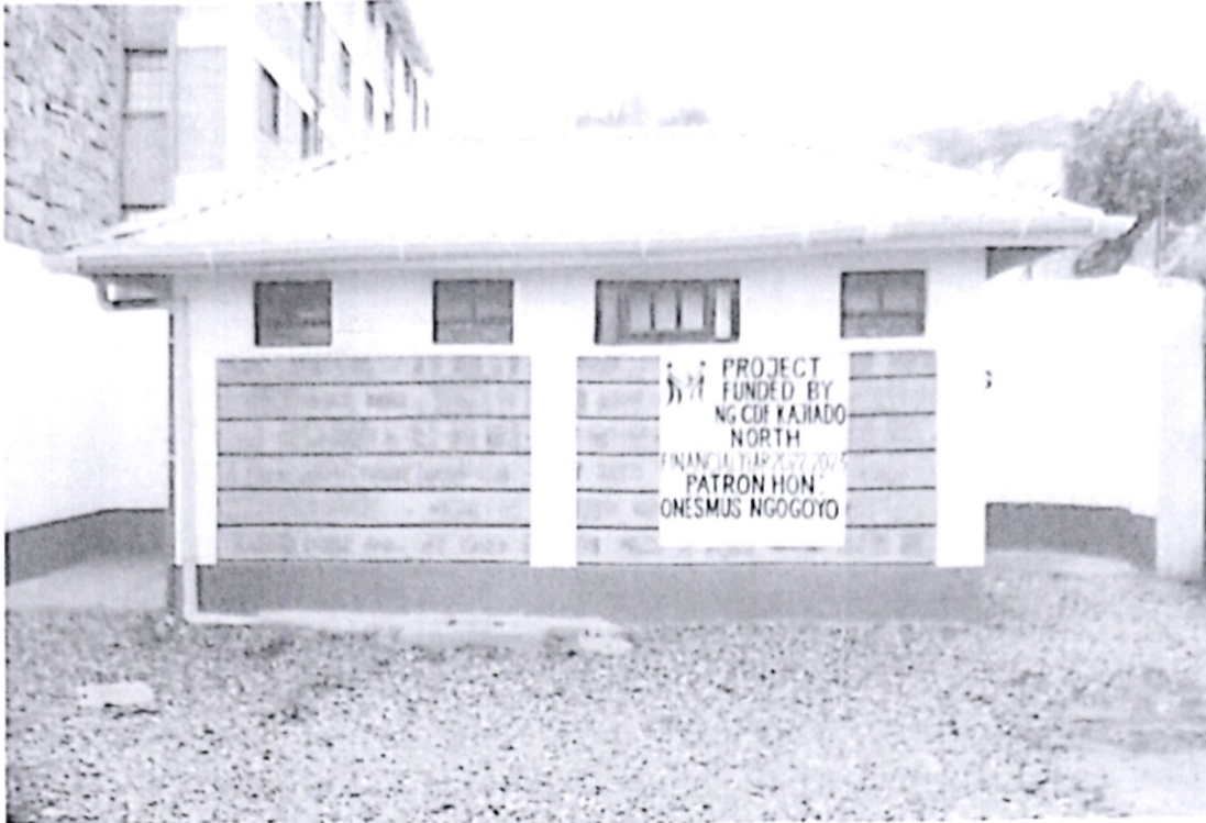
Toilet block at Ongata Rongai Assistant Chiefs office (Hellena Road) Impact: The project has impacted the whole of Ongata Rongai Sub location, who are able to receive national government and other services at the facility.
