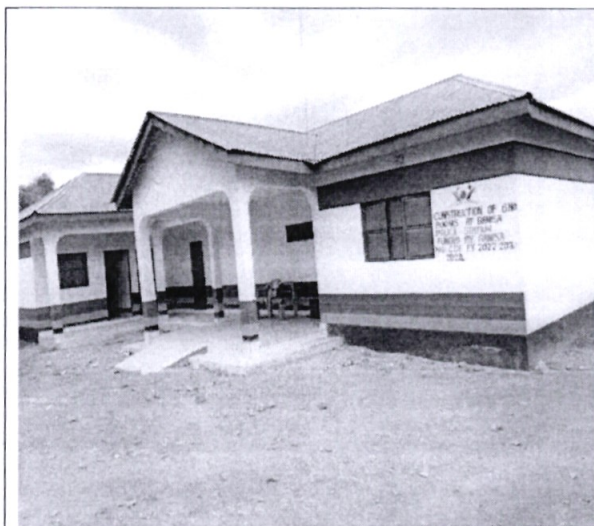
Banisa Police Administration Office newly built and in use. This has enhanced service delivery.
