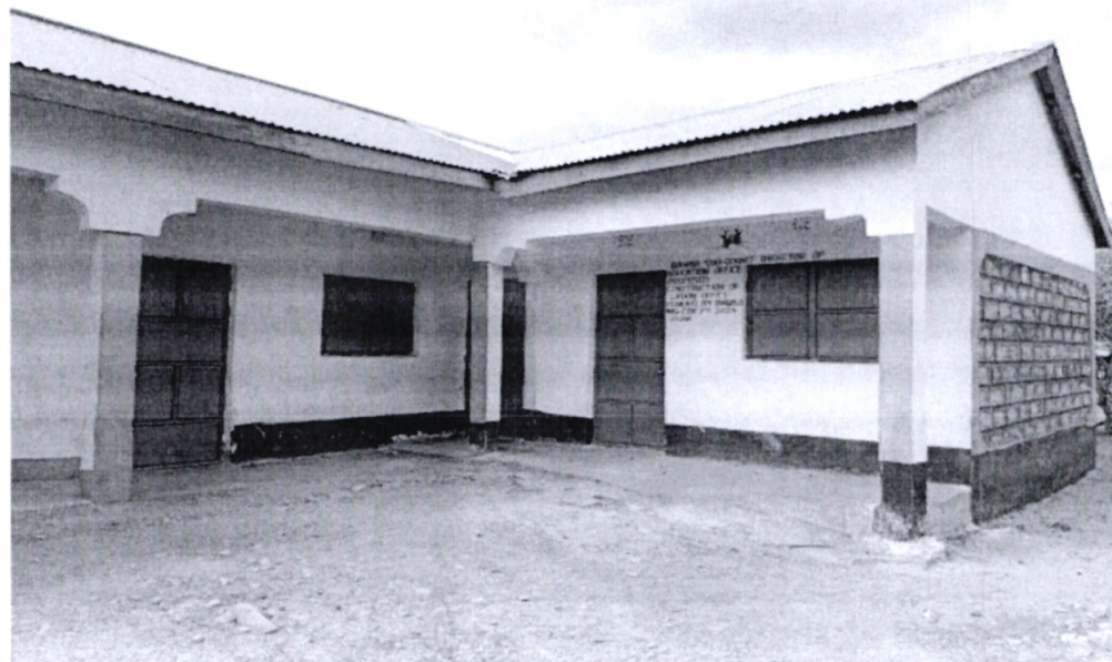
Banisa Sub County Director of Education has now a new office courtesy of Banissa NG-CDF. This has led to improvement in service delivery
