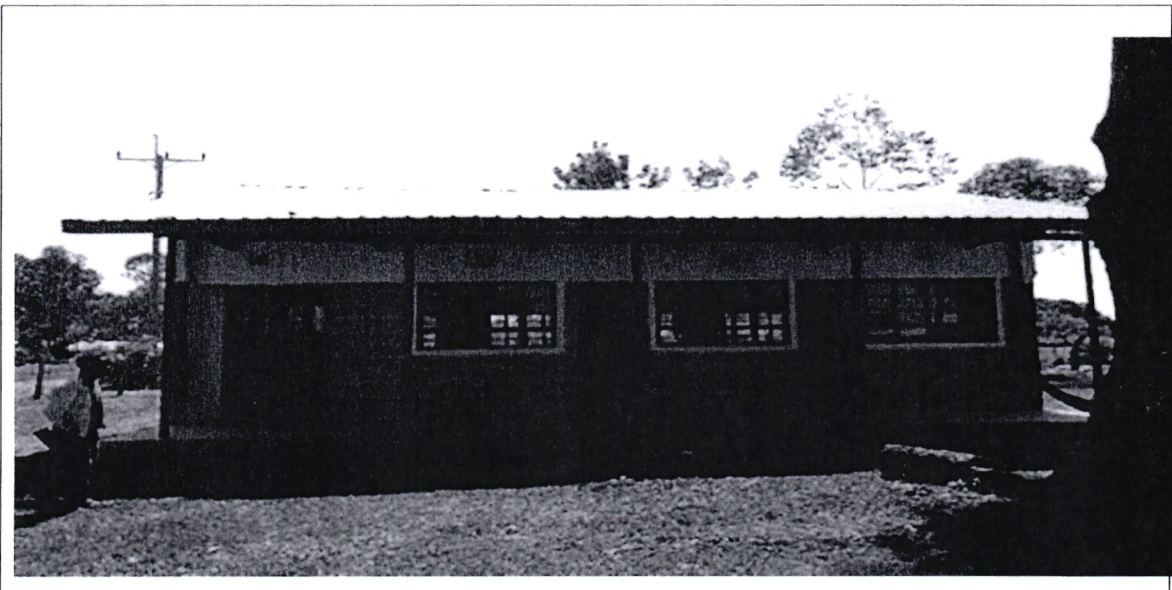
Figure 1: Newly constructed ECDE Classroom at Bwaliro Primary School in Busia County
