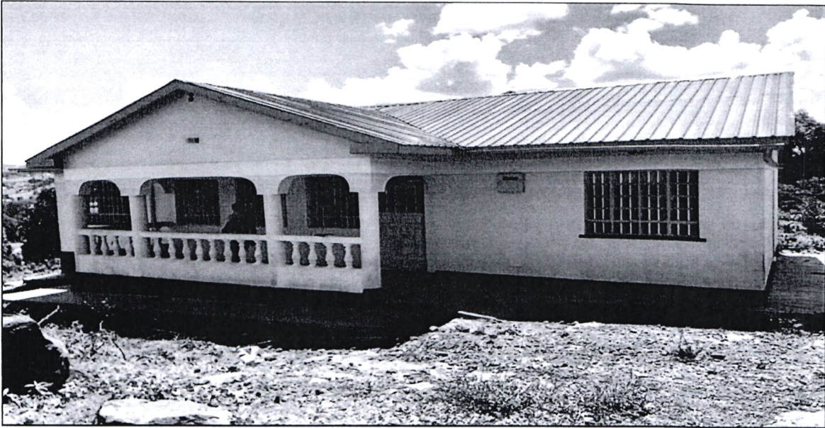
Figure 3: Newly constructed Got Agak Dispensary in Homa Bay County
