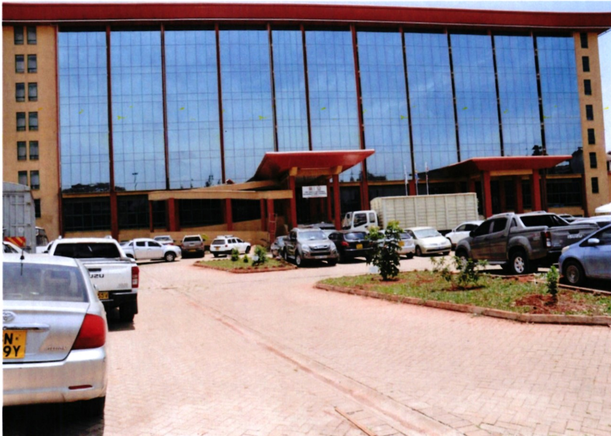
A view of New Mitihani House project
