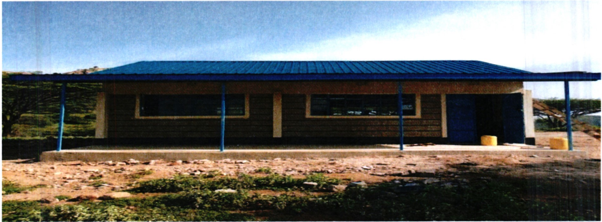
One of our CSR projects: ECDE Classroom at Nkorika Primary School in Oldonyiro. In addition to this, the Company also put up an additional ECDE classroom at Lturot Primary School, fences at Raap and Tuale Primary Schools as well as a dormitory and dining hall at Oldonyiro Secondary School.
