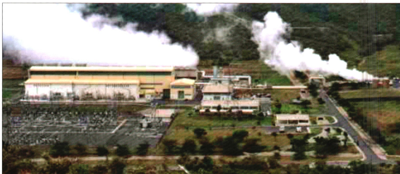
Olkaria geothermal power plant
