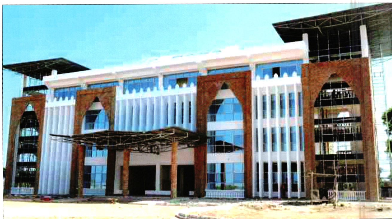
Lamu port office block nearing completion
