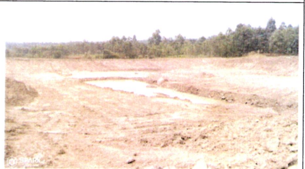
Changara Water pan excavation in progress
