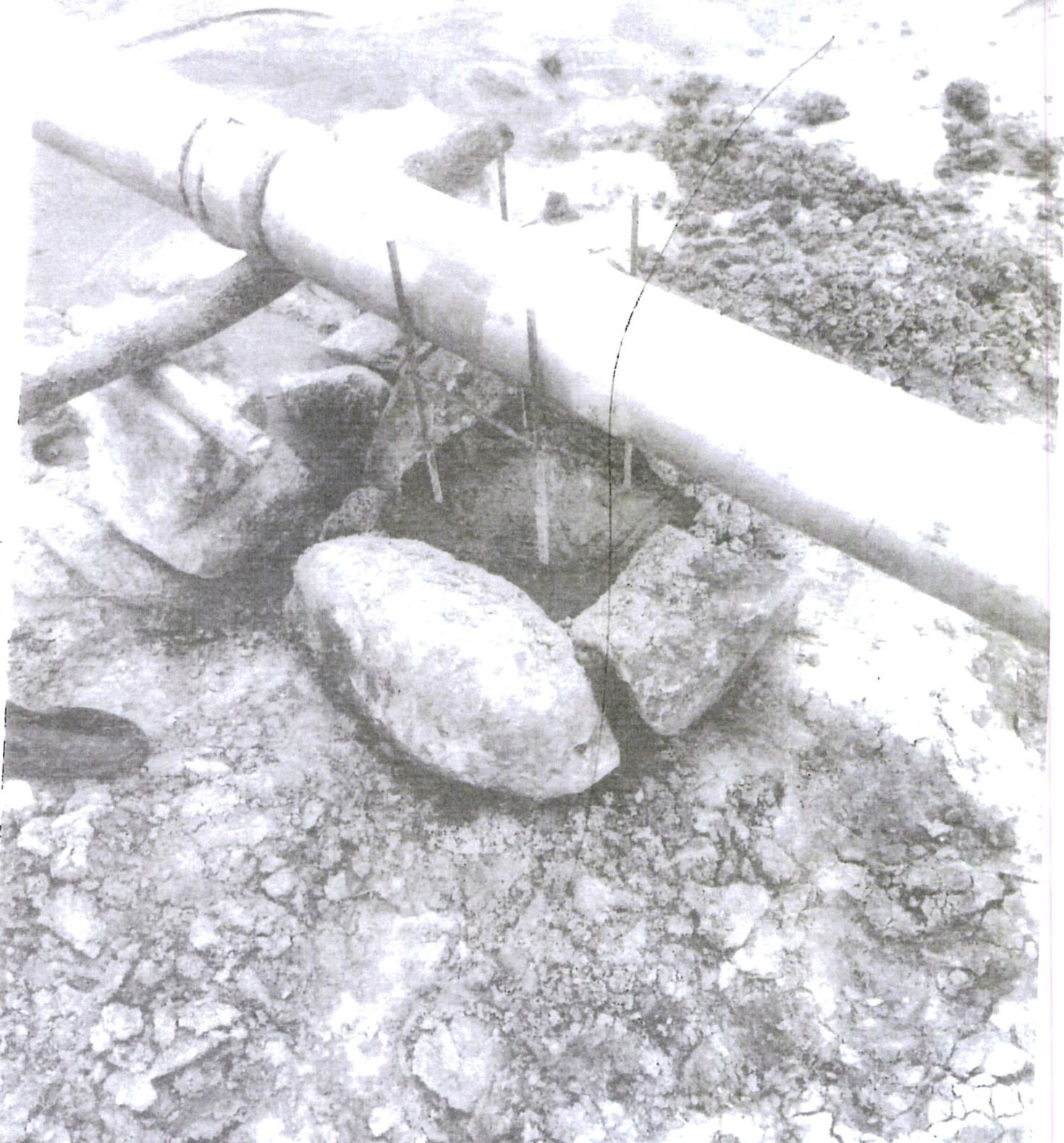
CASTING OF LAND PIPES
