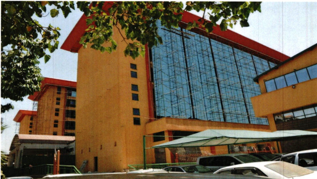
The New Mitihani House (Ongoing Project)
