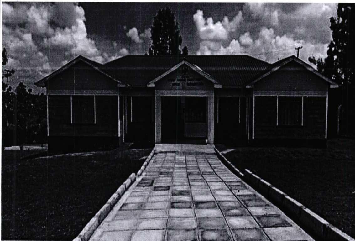
Saboti NGCDF Office, F/Y 2019-2020, Construction of office Impact: improved service delivery to the public
