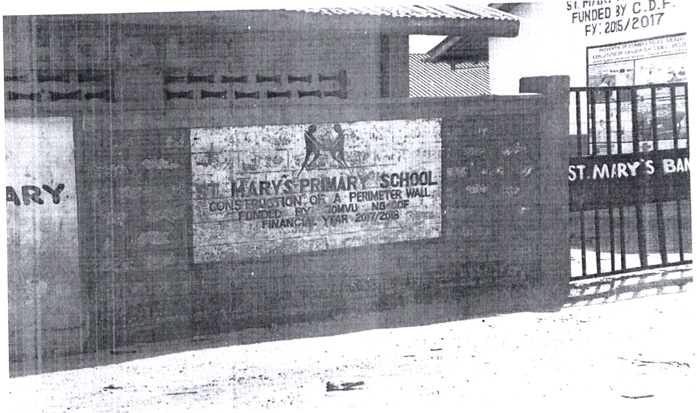
St. Mary's Primary School perimeter wall- complete
