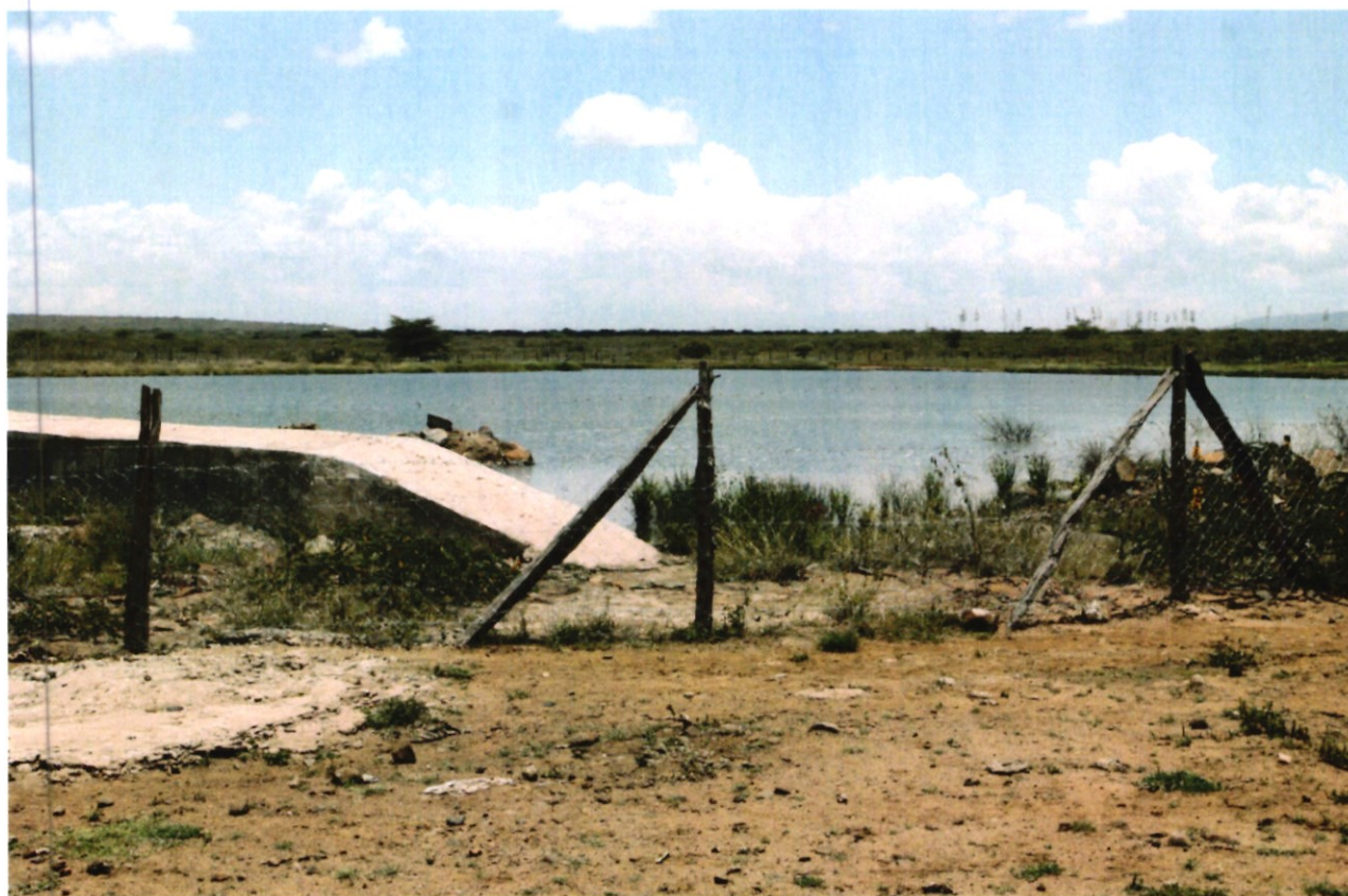
Lemmsiguyoi Weir Dam , Samburu County
