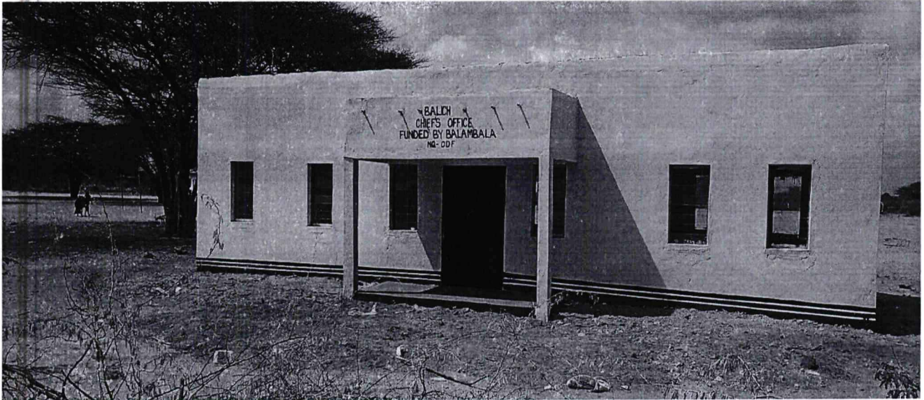
Balich Chiefs office – construction of chiefs office
