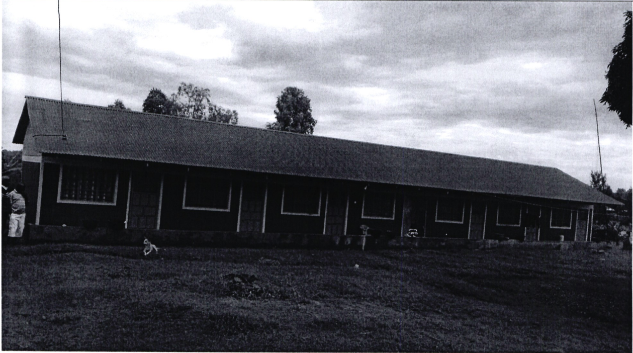
KITUTU CHACHE SOUTH NG CDF PROJECT-7 UNITS OF STAFF HOUSES CONSTRUCTED BY NG-CDF AT RUGA AP. LINE
