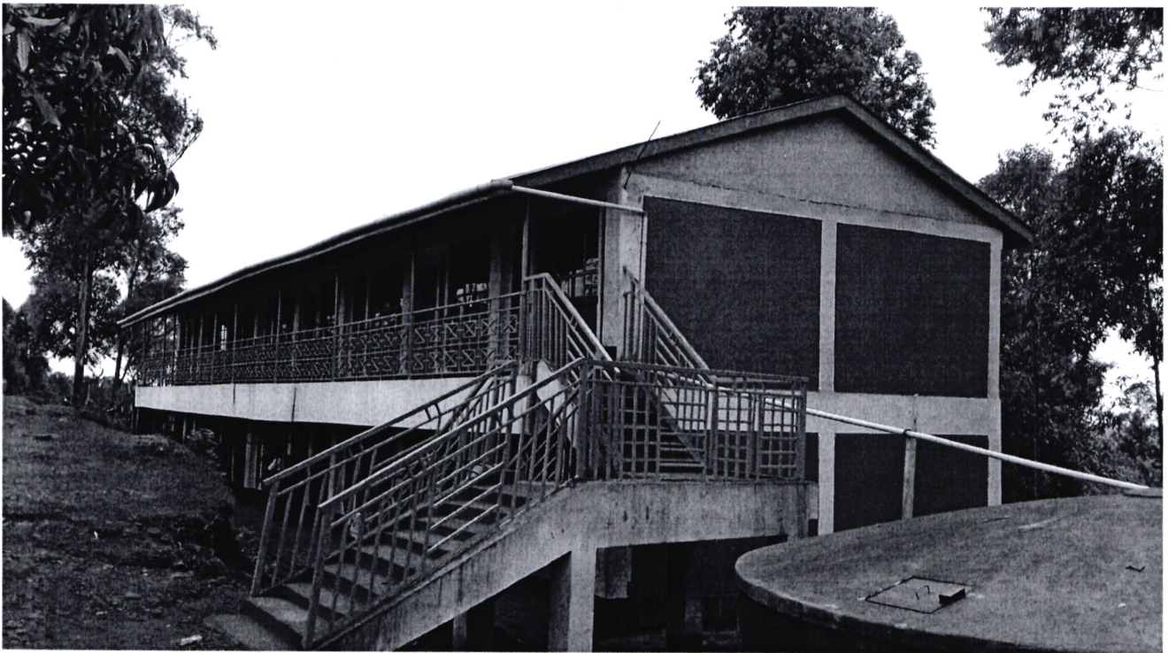
KITUTU CHACHE SOUTH NG CDF PROJECT-8 CLASSROOMS CONSTRUCTED BY NG-CDF AT KIANYABINGE PRIMARY SCHOOL
