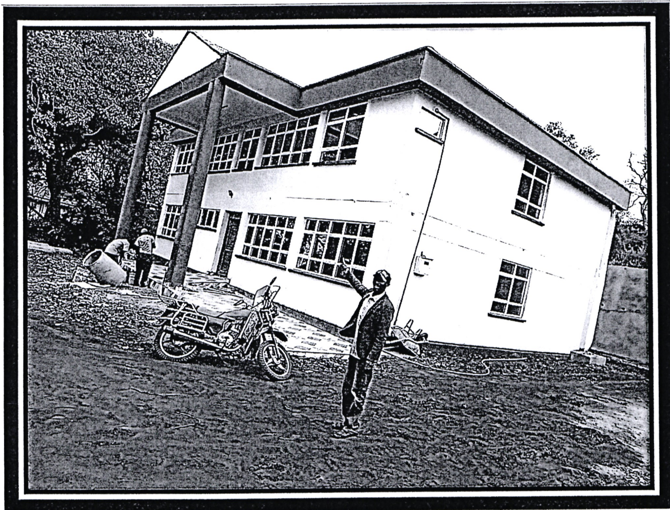
NGCDF Office complex
