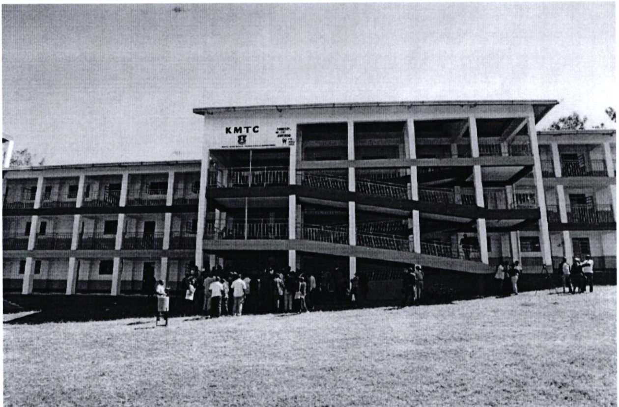
FY 2022-2023: Completed Awendo KMTC which is in Use
