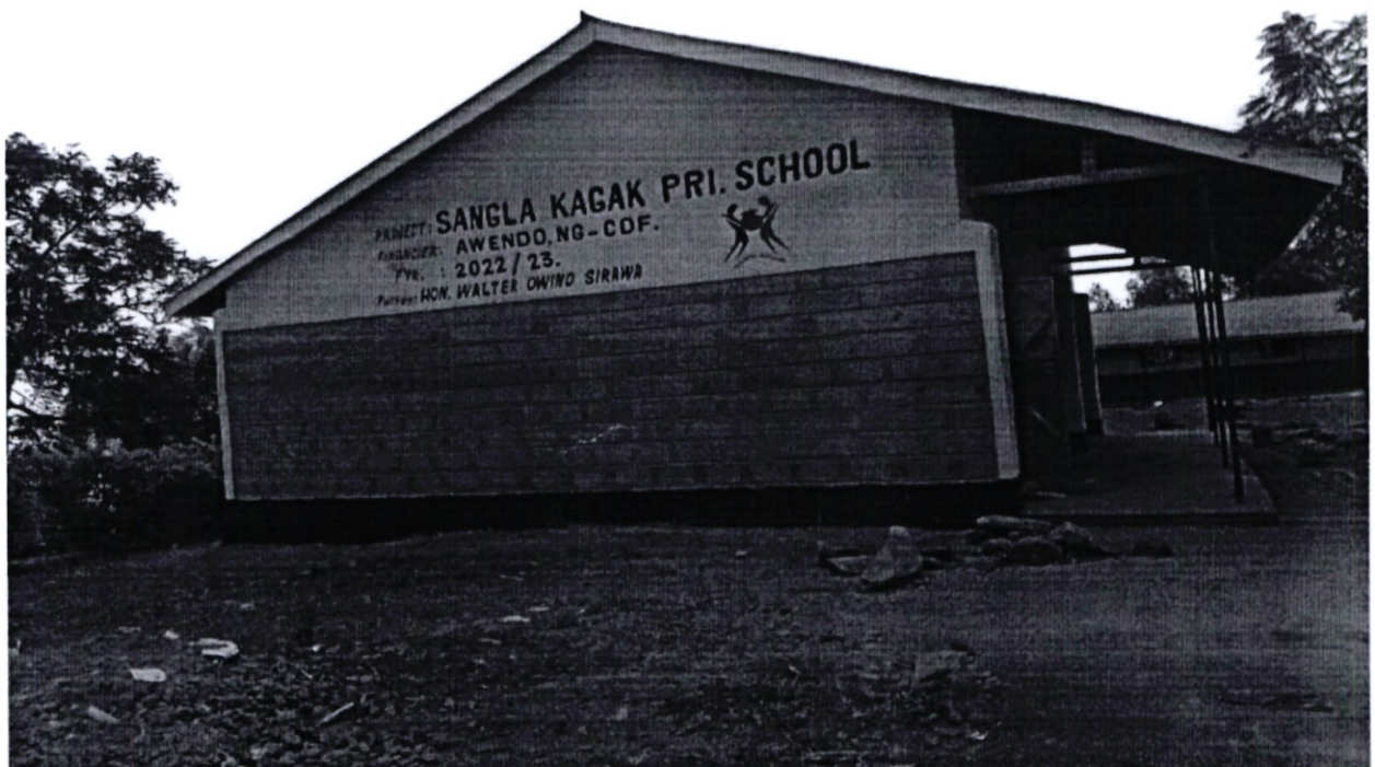
FY 2022-2023: Completed classroom at Sangla Kagak
