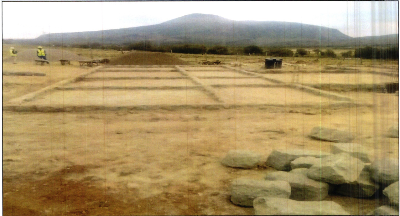
Narasha dispensary at foundational stage
