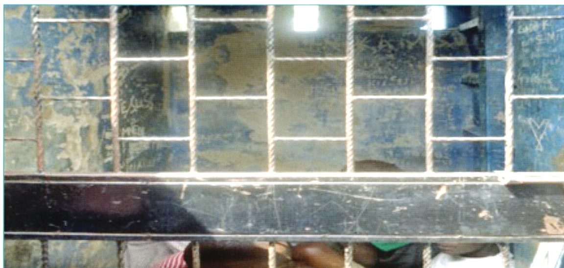
Extremely small cell at Kiembeni Police Station in Mombasa County
