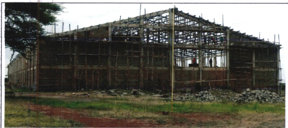
Oloitokitok Agro-Processing project super structure under construction
