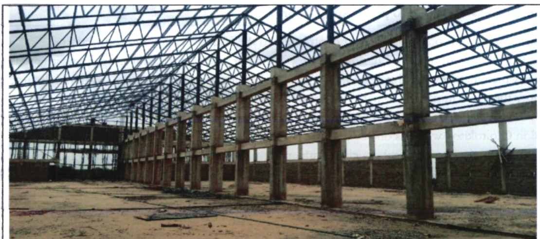
Steel structure ready for roofing.
