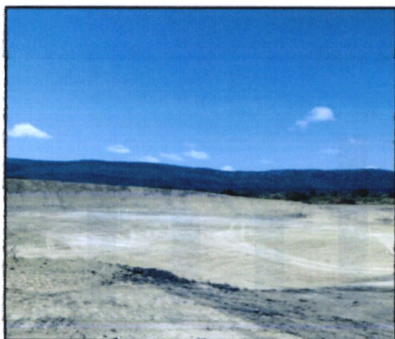
Completed Nkineji water pan
