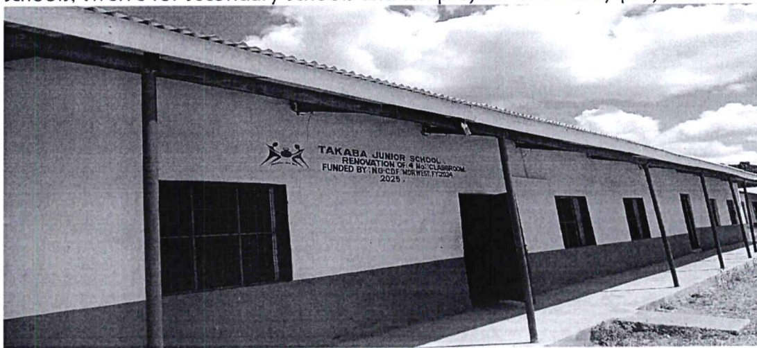
Renovation of four (4) classrooms at takaba primary and junior secondary school
