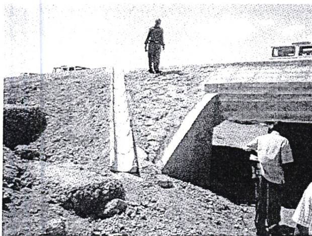
Outlet to 4m X 2 m Box Culvert
