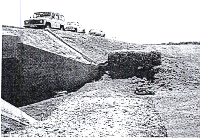
Inlet to 4m X 2 m Box Culvert
