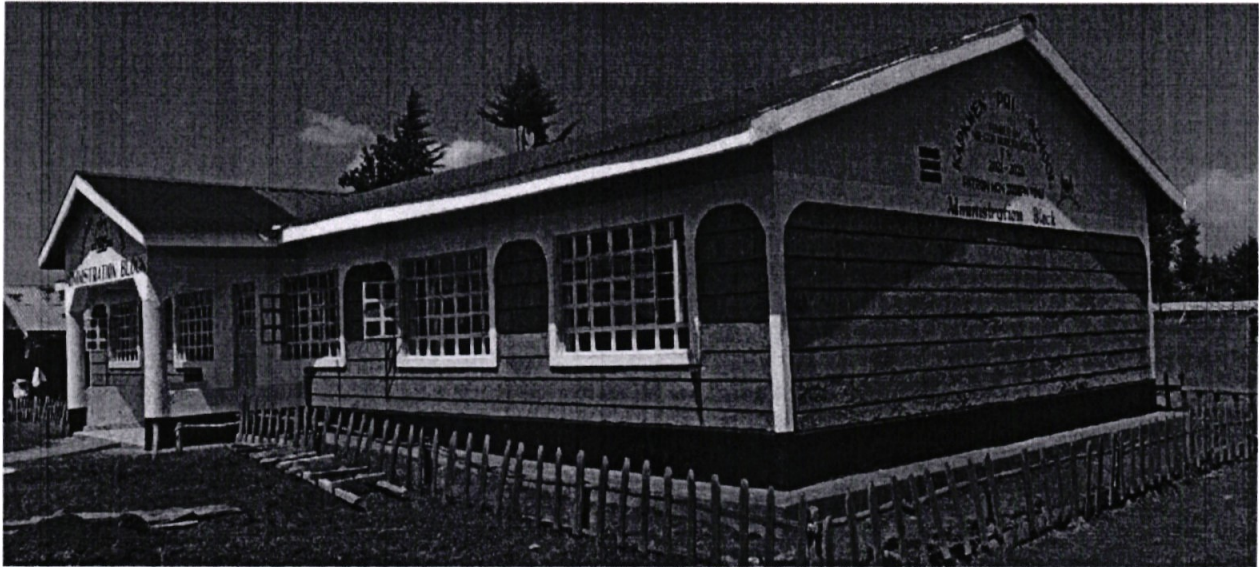
Kapkwen Primary School: Construction of Six Office Administration Block
