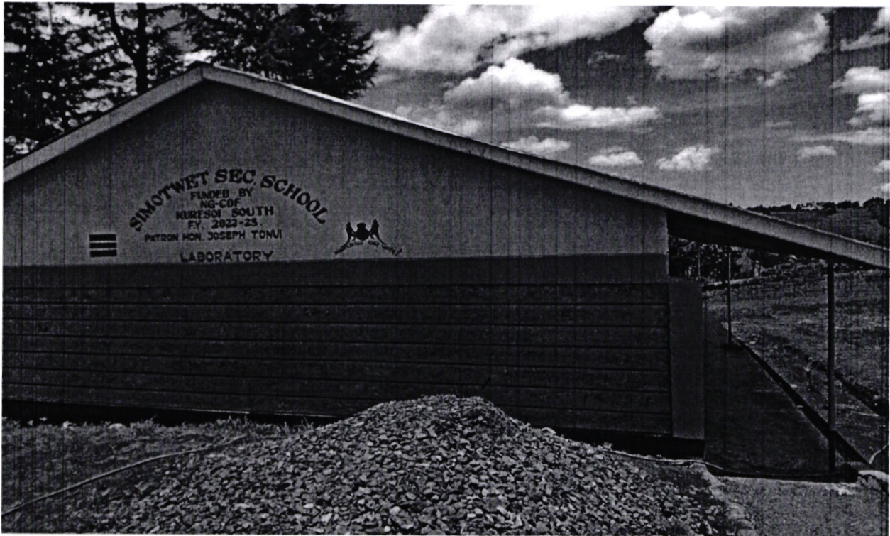
Simotwet Secondary School: Construction of 45 student capacity laboratory
