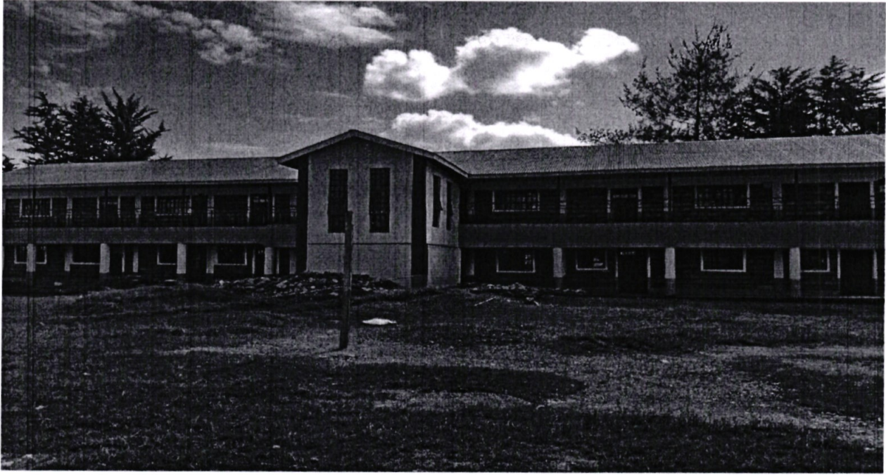
Ketitui Central Primary School: Renovation to completion of 10 Classrooms
