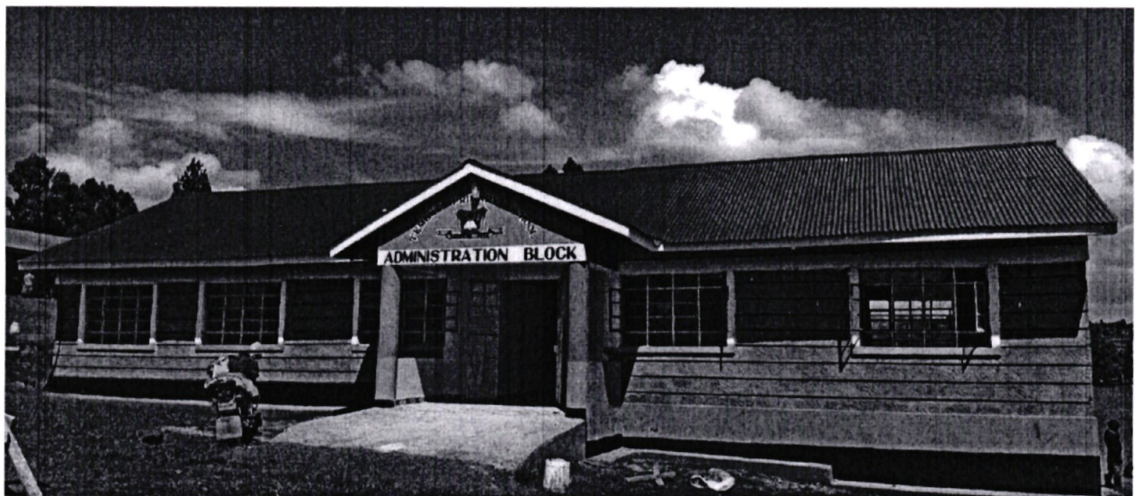
Tembwo Primary School: Construction of Six Office Administration Block
