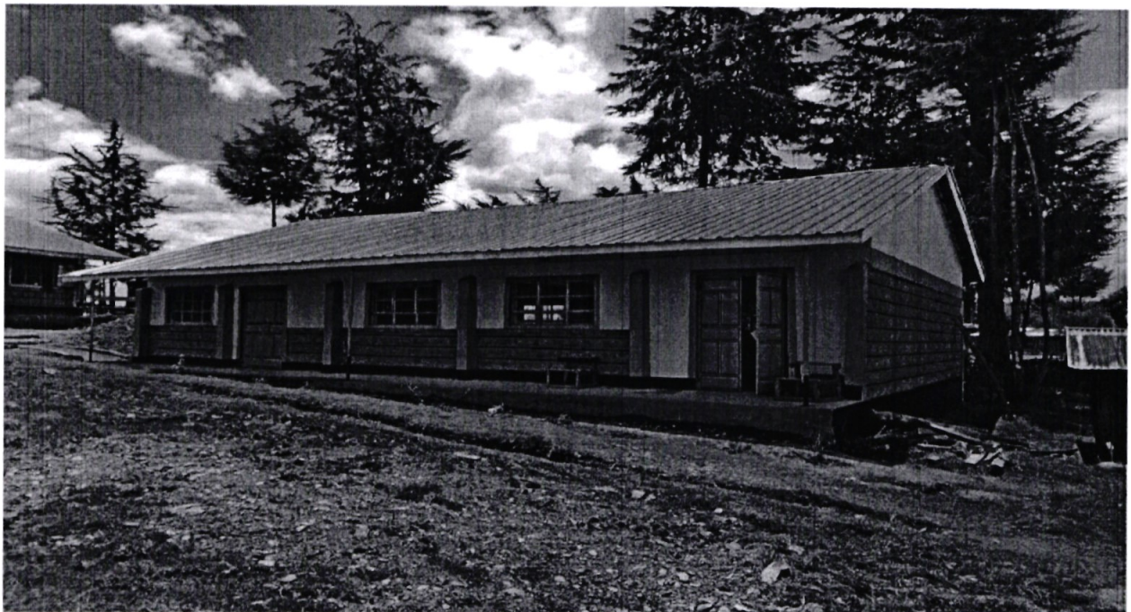
Simotwet Secondary School: Construction of 45 student capacity laboratory
