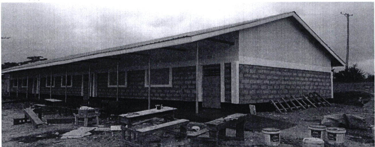
Cheparor Primary School Construction of Classes to Completion B.
