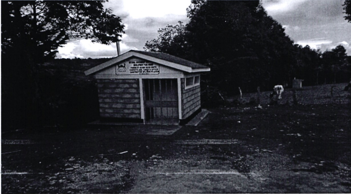
Chororget Primary school -Emergency toilet construction
