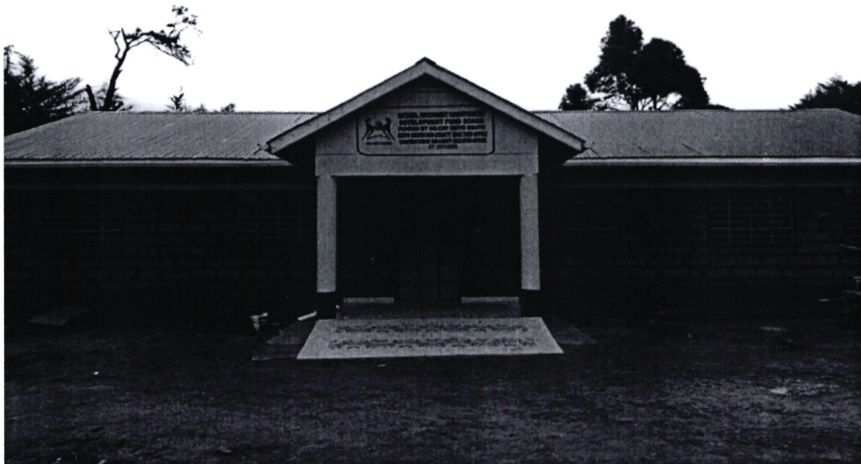
Keiyo South Ministry of Education -Construction of office
