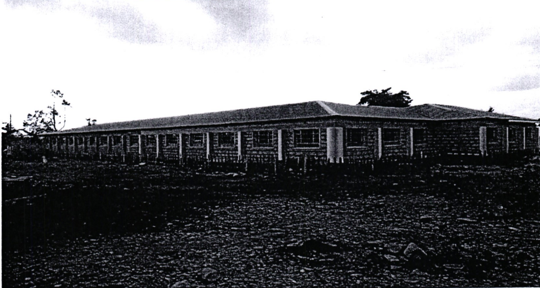
Kilingot Primary School – Construction of Eight Classrooms
