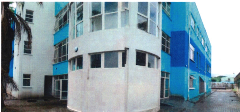
100% complete External View Day care center
