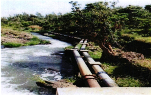
Twin Conveyance at Nithi Kari irrigation project
