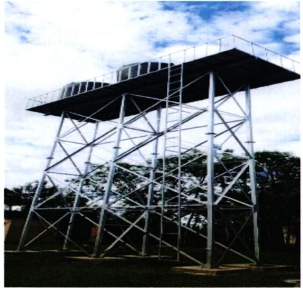
Elevated tank tower in Rapora Mixed Secondary School
