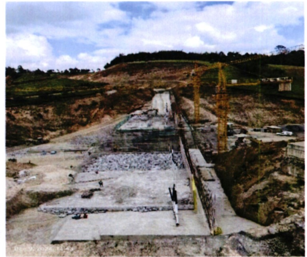
Cyclopean Dam Embarkment in Muruny (Siyoi) Dam, Kapenguria water project
