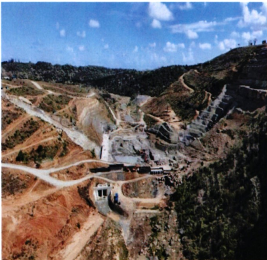
Embarkment wall in Sugutek Earth Dam
