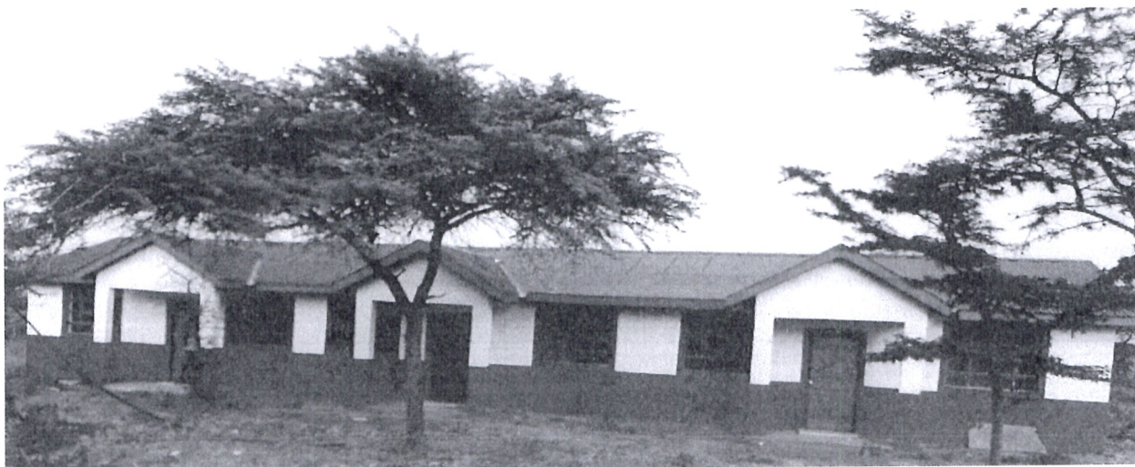
Figure 2: Kulal Girls Secondary School-Construction of Three unit staff quarters to completion
