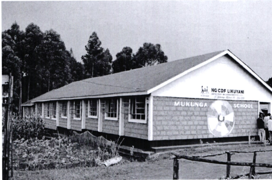
2 Classes with an Administration Block at Mukunga Comprehensive School-Kongoni ward
