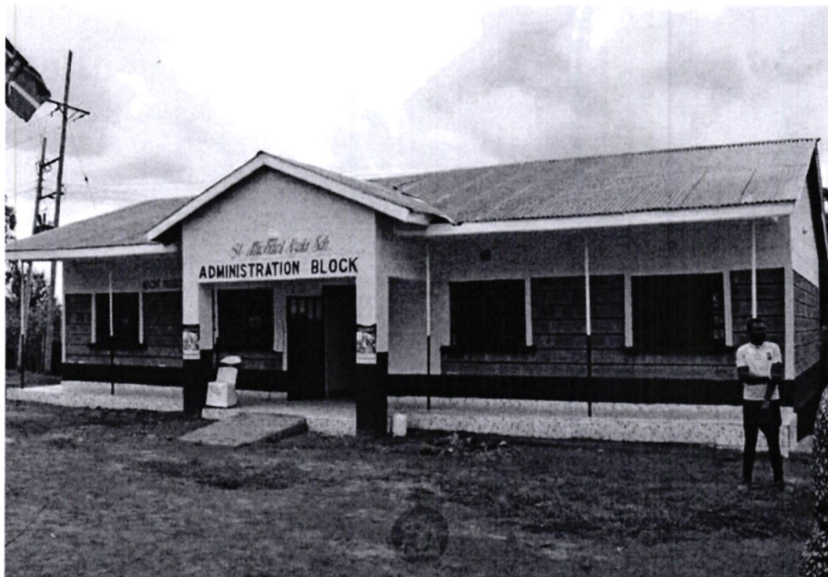
An Administration Block at St. Michael Nzoia Comprehensive School
