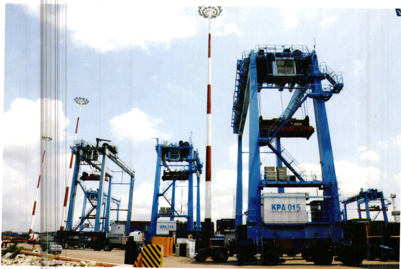
Mombasa Port Berths
