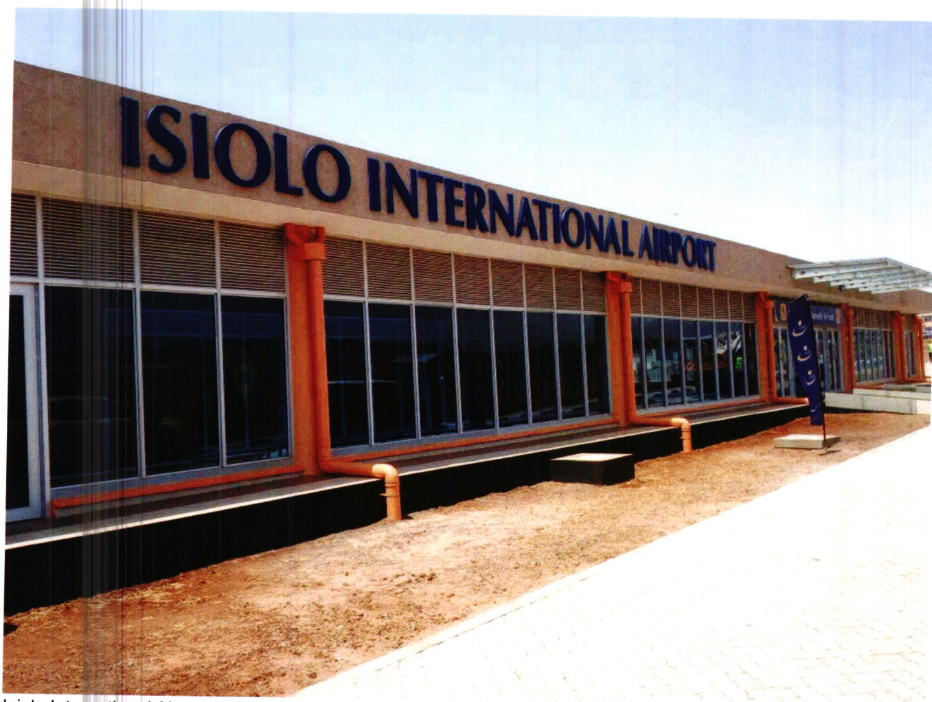
Isiolo International Airport under construction
