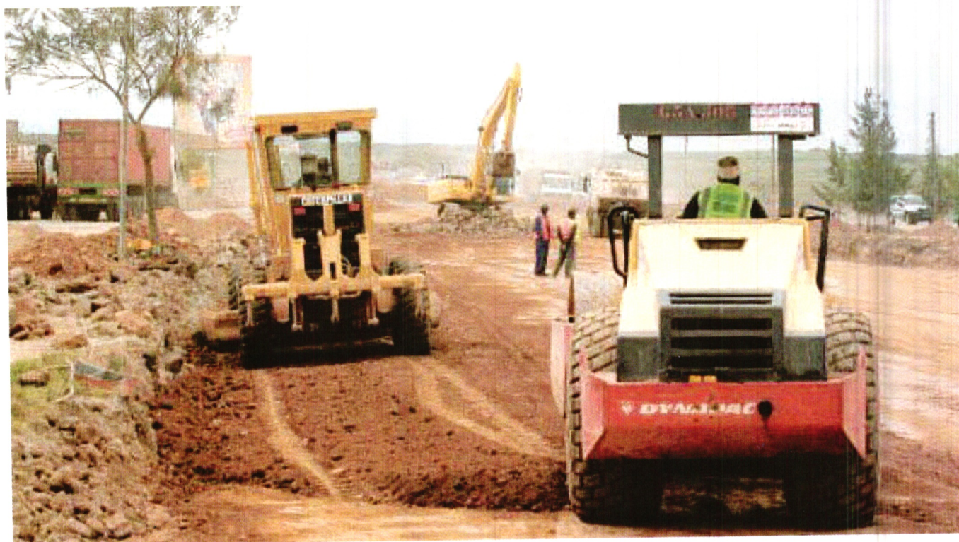
Eldoret-Turkana road under construction
