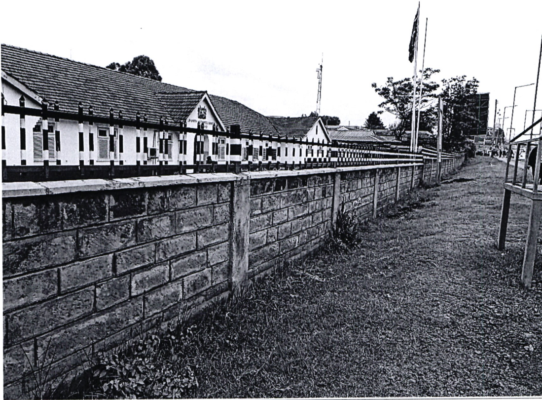
DCC office perimeter fence FY 19/20
