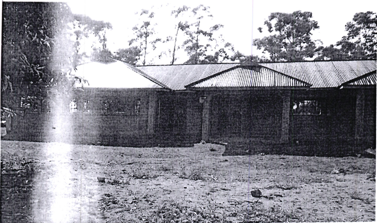
Above: mabera Resource Center funded in security sector
