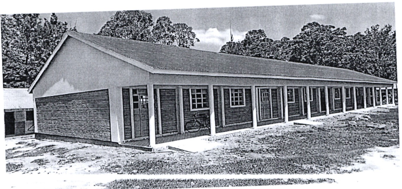
Figure 1: Kamunoit Primary School – Construction of 4 no. classrooms
