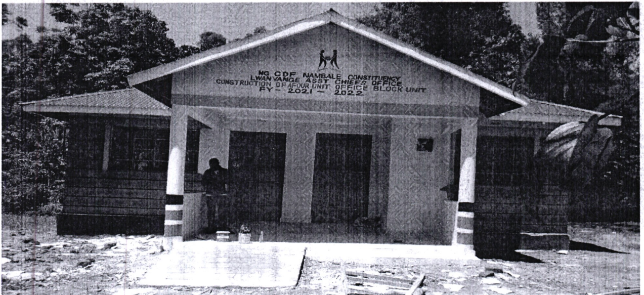
Fig4. Lwanyange Assistant Chief's Office-Construction of a Four Unit Office Block
