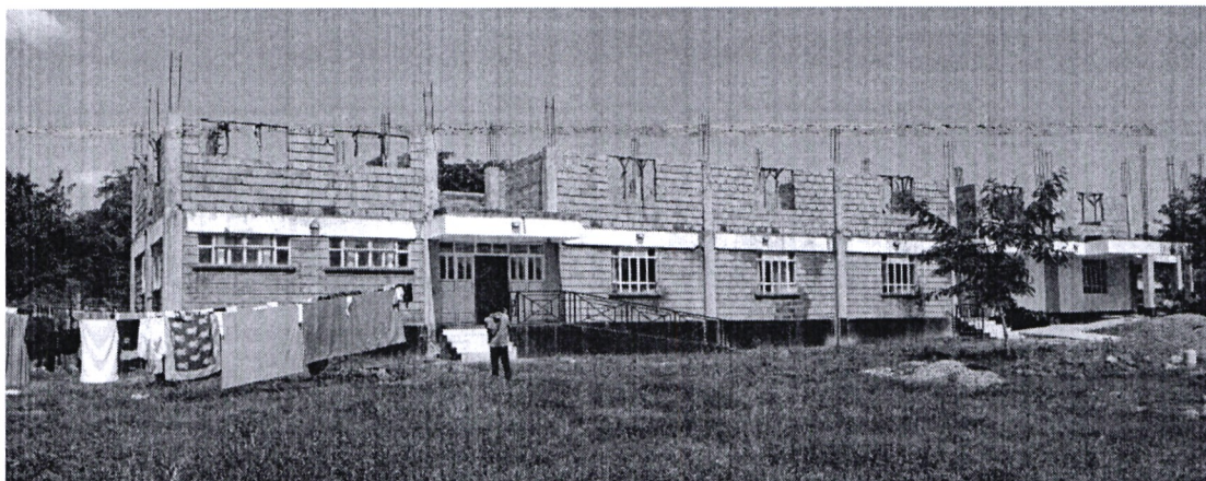
Fig1: St. Pauls Elwanikha Girls Secondary School-Construction of 2 Storey 300 Capacity Dormitory
