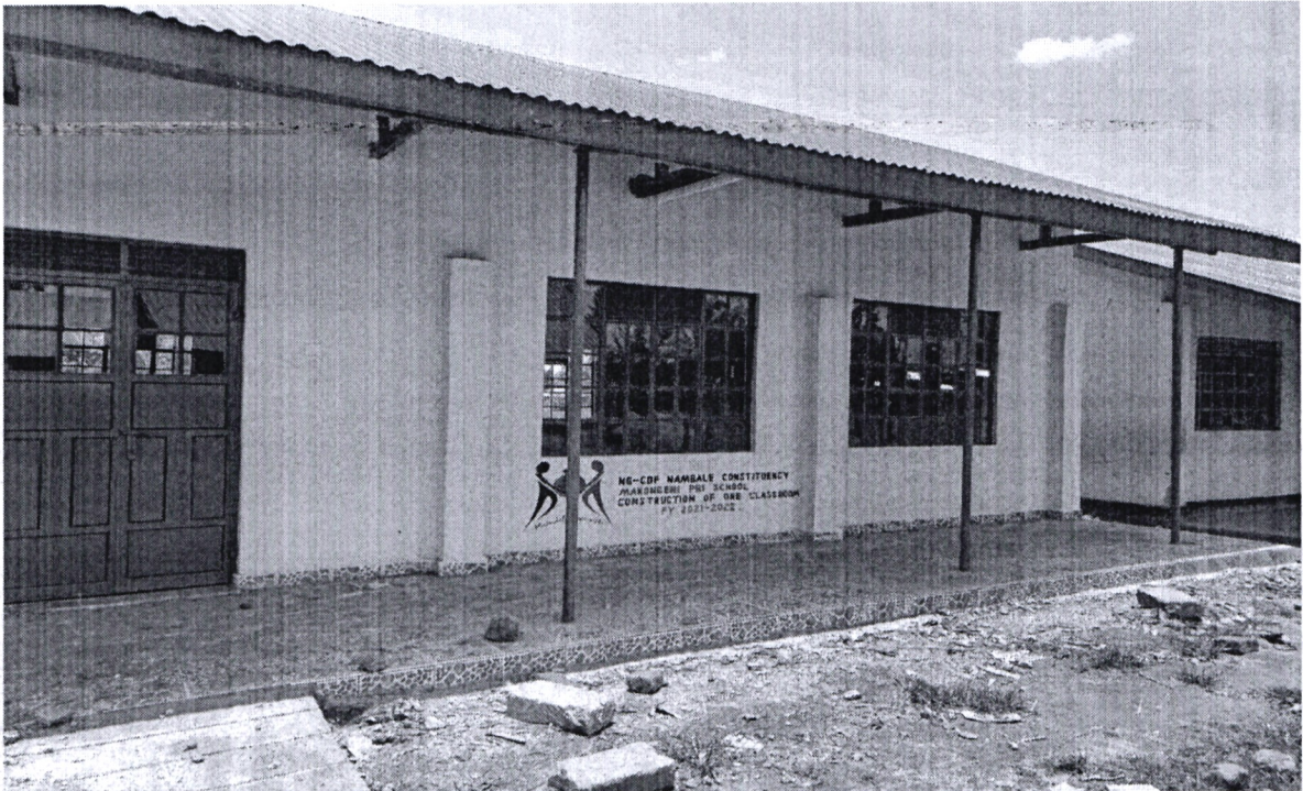
Fig5.Makongeni Primary-Construction of One Classroom
