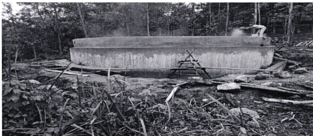
Structures that made up Chebululu Spring Water Project
