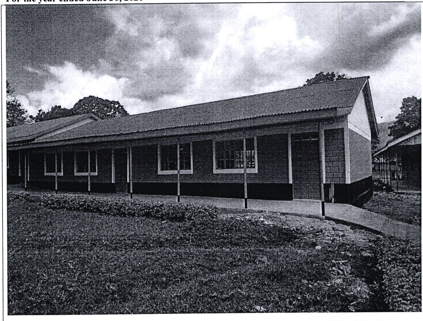
Fig. 3: Chepareria Mixed Secondary School, ongoing completion of 2 Classrooms
