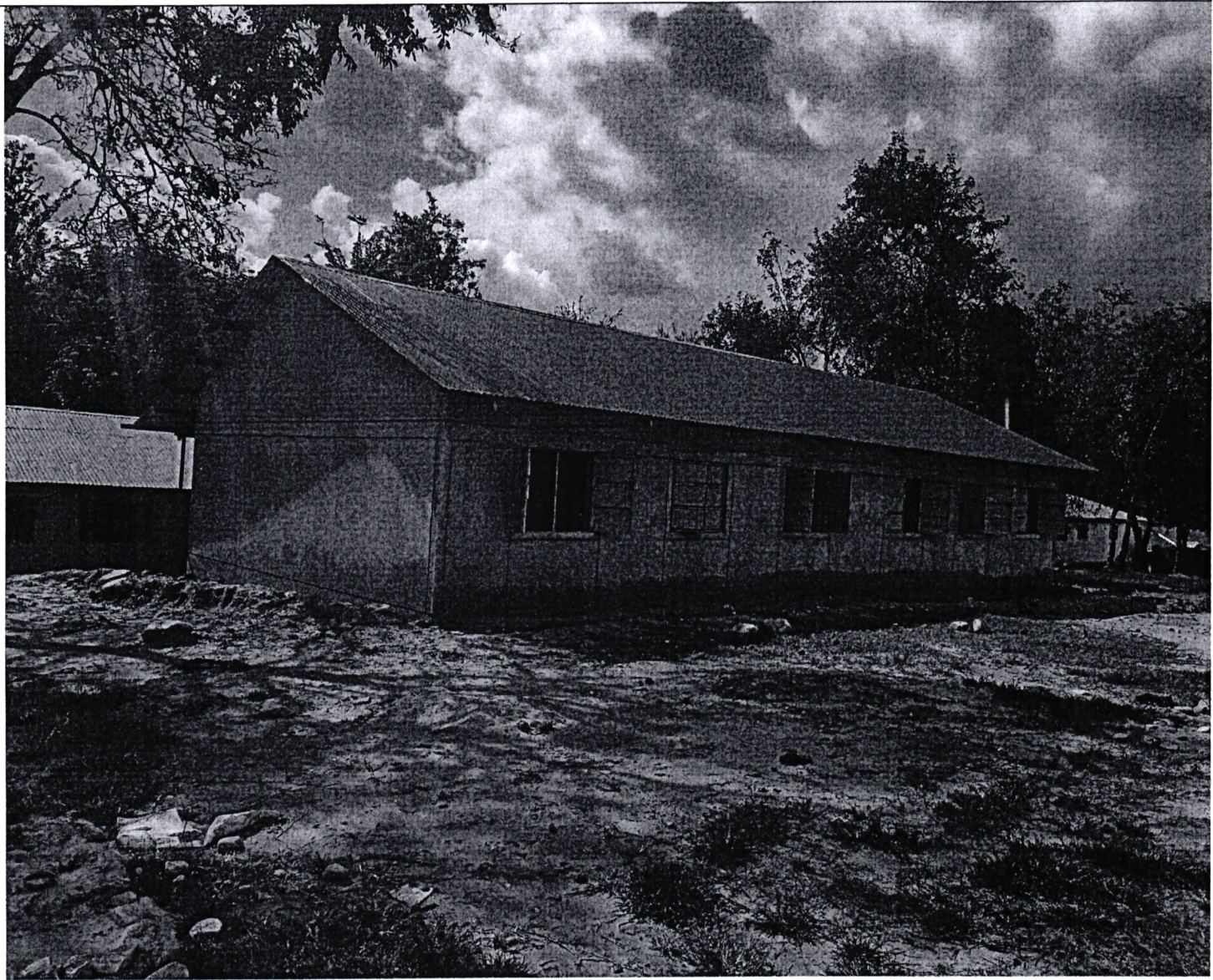
Fig. 2: Chelombai Primary School, 2 Classrooms under Construction
