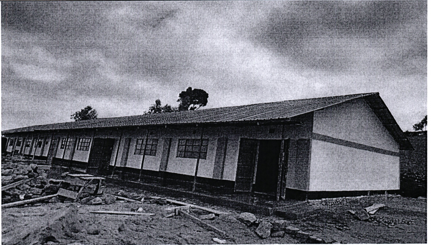
Fig. 4: St. Paul Lomuke Secondary school, 2 classrooms under construction
