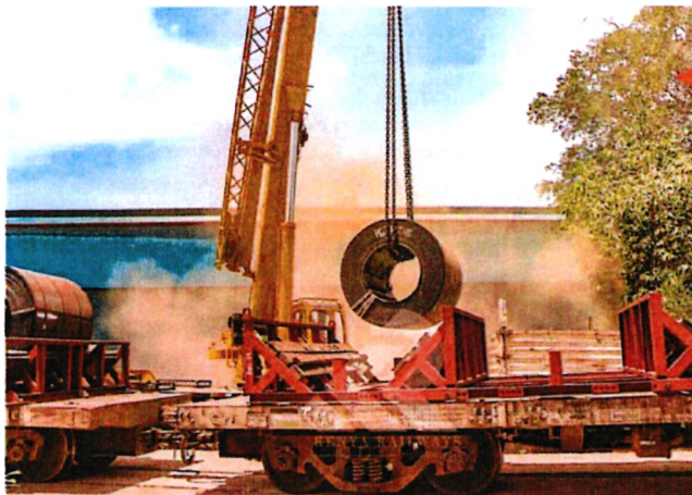
Offloading of hot rolled coils (HRC) at Devki Athi River plant, following the construction of an MGR rail siding to the plant. Railway sidings enable us offer last-mile services to our customers. What are you transporting
