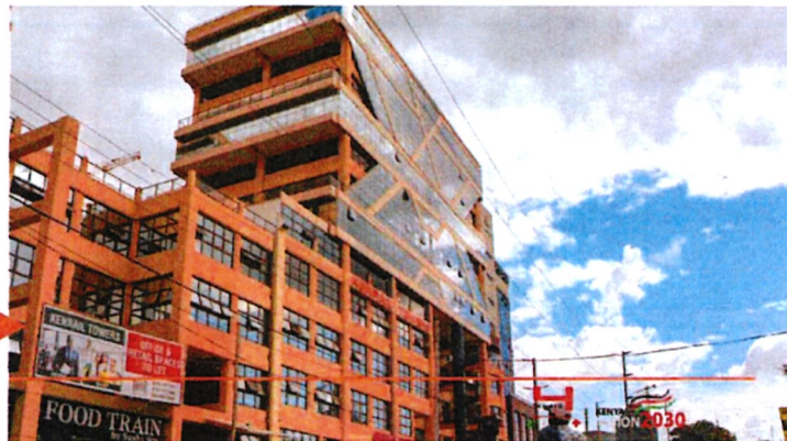
Kenrail Towers in Westlands Nairobi. It offers modern office space in prime location.
