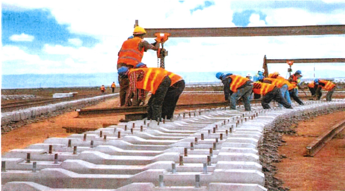
Construction of Naivasha - Longonot
