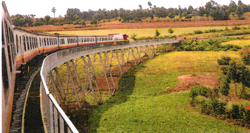
Nanyuki bound passenger train navigating over one of the rehabilitated bridges. Nanyuki boasts of its scenic landscapes and the magnificent Mt. Kenya, which is a favourite spot for hikers. Since the rehabilitation of the Nairobi- Nanyuki railway line, we have transported over 45,000 passengers to Nanyuki.
