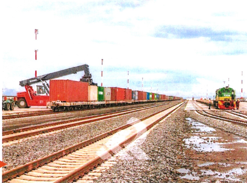
SGR Cargo Train being offloaded at Naivasha ICD. SGR now serves the regional market needs by safety and reliably transporting cargo from the port of Mombasa.
